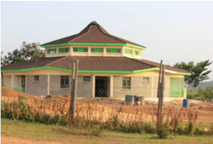
The hospital initially will serve as a joint outpatient clinic and inpatient short-stay, 10-bed pediatric ward.
